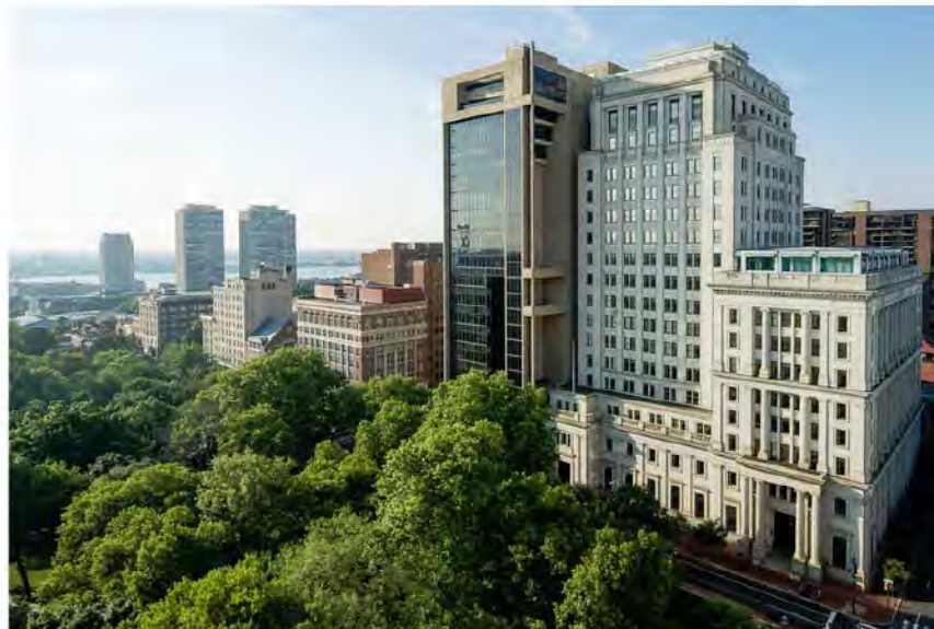
Penn Mutual Building, Philadelphia, PA
